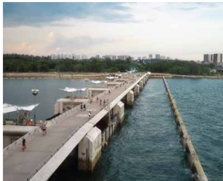
The Marina Barrage is a dam built across the 350m-wide Marina Channel, and part of a comprehensive flood control scheme to alleviate flooding in downtown Singapore.
