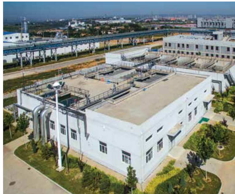
Sembcorp's plant in Changzhi, China, utilises a zero liquid discharge model. (Photo courtesy of Sembcorp Utilities)
