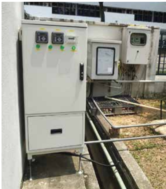
EnviroSens' i2BioS continuously monitors water quality and automatically collects samples when toxicity levels rise above safe levels. (Photo courtesy of EnviroSens)
